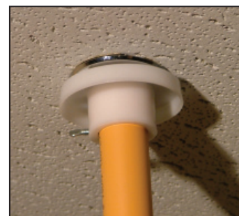
Figure 5: Correct use of the Cover Installer Tool
