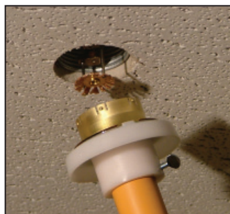
Figure 4: Use the Cover Installer Tool to Install the Mirage® Concealed Cover Plate.
