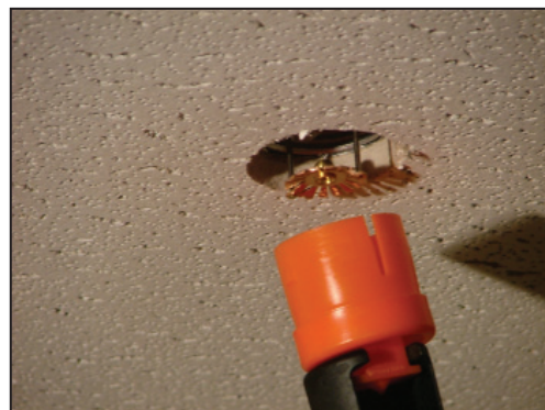
Figure 2: Use Sprinkler Wrench 14031 to remove the protective sprinkler cap.
