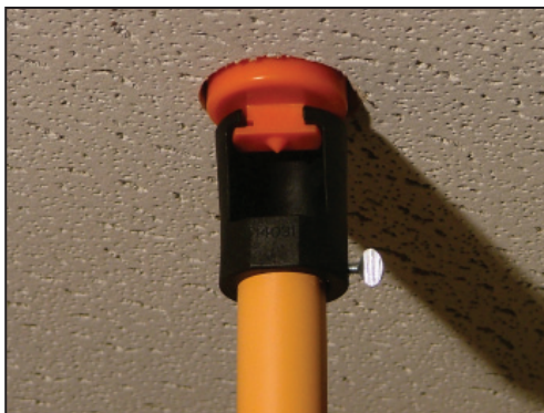
Figure 1: Attach Sprinkler Wrench 14031 onto a length of 1" diameter CPVC pipe
