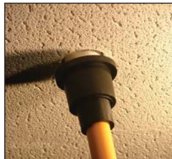
Figure 3: Press the escutcheon cup onto the adapter until the flanges touch the ceiling.
