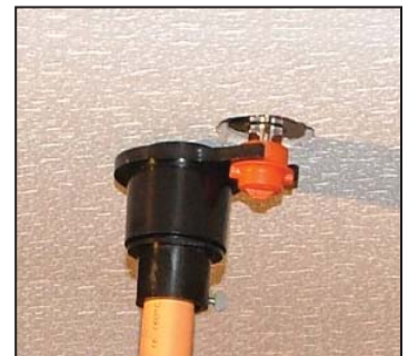
Figure 4: With the tool attached to the end of the CPVC pipe, place it onto the sprinkler cap and pull to remove the cap from the sprinkler.
