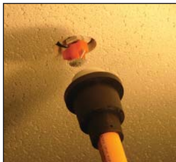
Figure 2: Place a Model E-1 or F-1 escutcheon cup in the installer tool and use the tool to install the cup onto the sprinkler and adapter.
