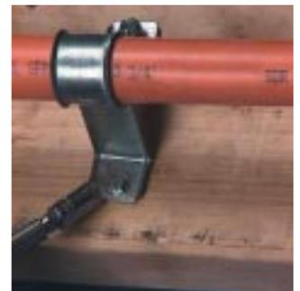
3. Fasten the strap to the wood surface using the two screws provided. (#10 x 1 hex washer head unslotted, self-tapping.)
