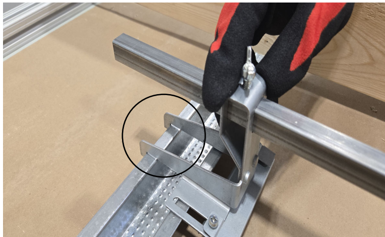
Figure – 2: Bracket Leg End Hook on Channel Edge
