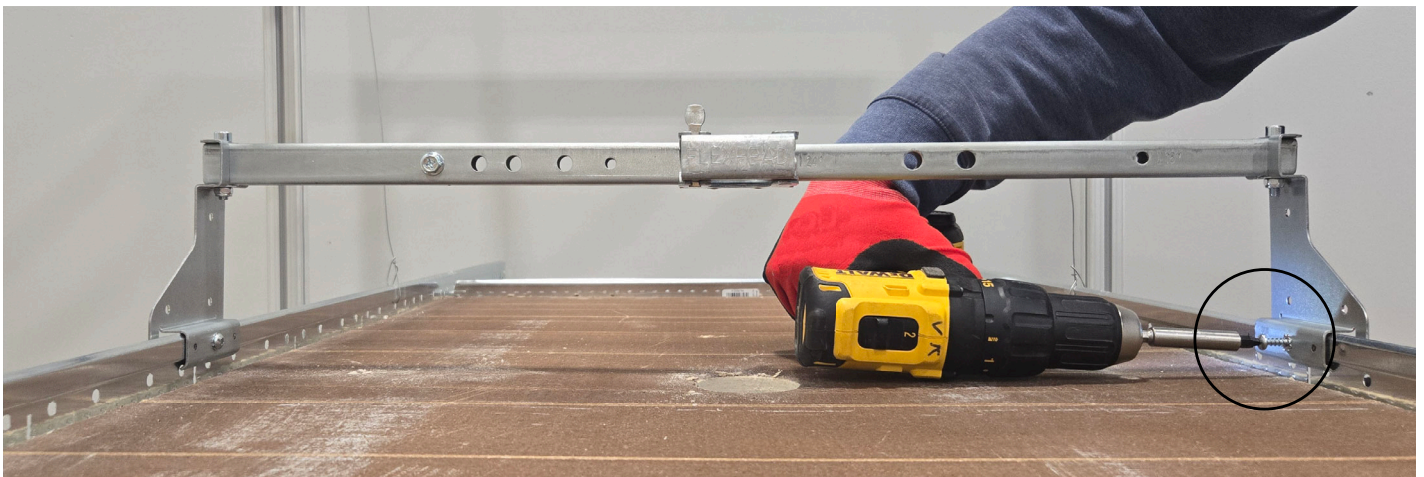
Figure – 2: Install Mounting Screws into T-Bar
