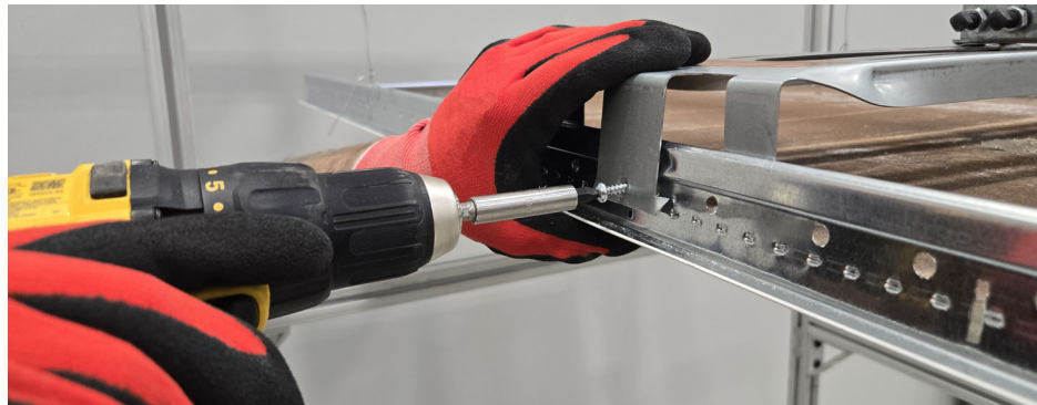
Figure – 2: Fasten Bracket onto T-Bar
