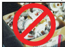
INCORRECT (Protective caps not in place)
